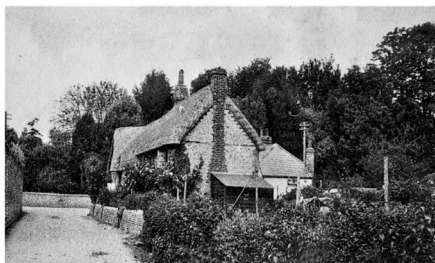
Hallidays, the cottages in Watery Lane, converted into a restaurant, which acquired a national reputation
